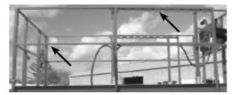
Figure 4.5 – Fall Restraint
