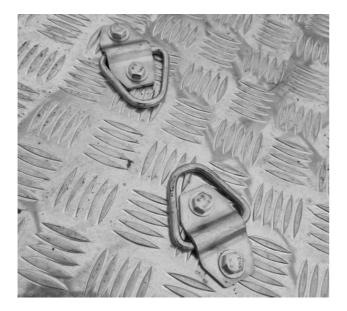
Figure 4.15 – Fall Restraint Points
